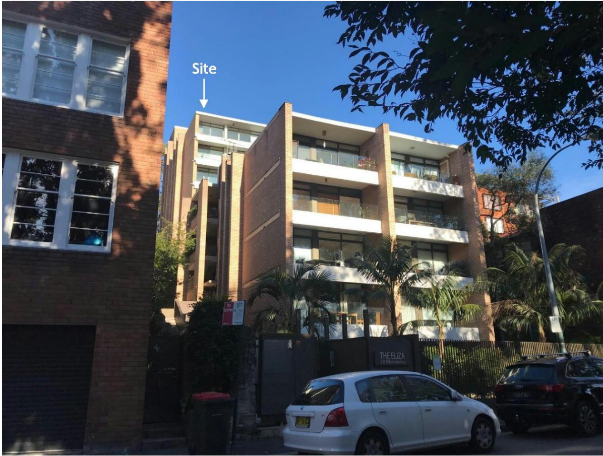
view of site from Billyard Avenue
