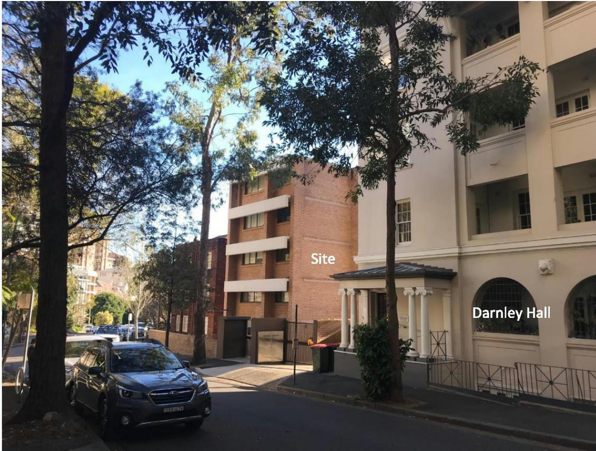
looking north along Onslow Avenue
